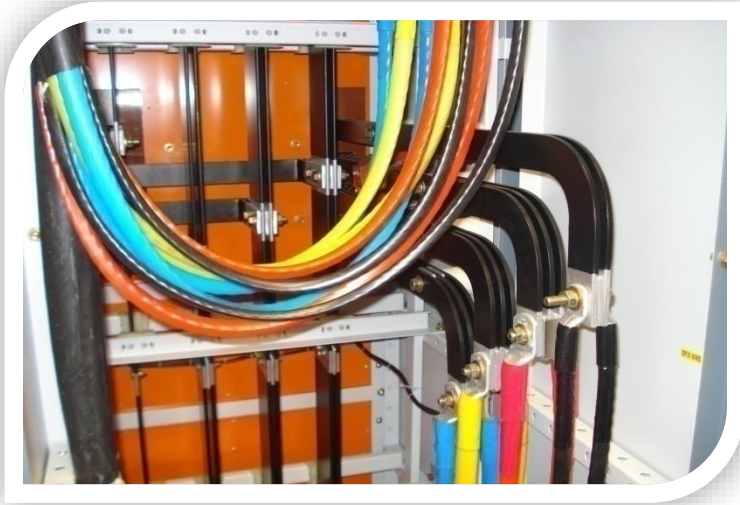
BUSBAR WITH EDGE BENDING
